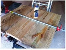
boards. Drill holes in the edges of the boards where they meet, then insert dowels into them and glue them in place with wood clue. Clamp and allow to dry for 24 hours.
