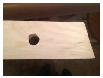
3. Flip your boards over to the other end (the top) and make a mark about 2" down from the top of each board, centered. Drill one hole in each board using the 1 1/4" drill bit. (This is where your top dowel will enter.)
