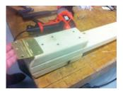
Step 13: Attach the hinges between the hip boards (F) and the torso board (E), making sure to test fit them first. Leave about a 1/4" between the F hip board and the H joint board, allowing the F board to fold down without being obstructed.
